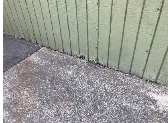
Worn siding (east side)
